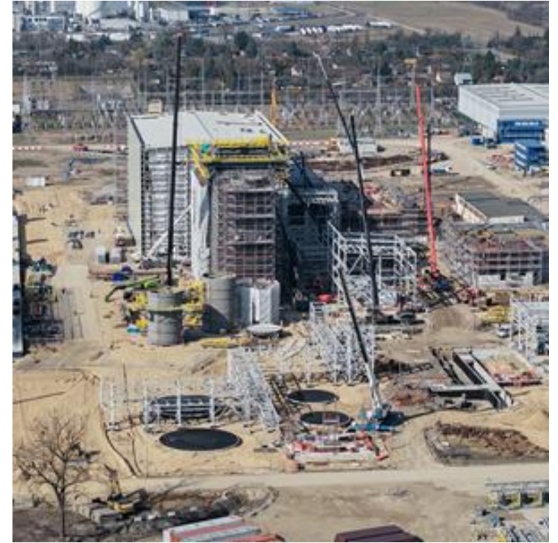
▲ CCGT unit construction site in Turek
