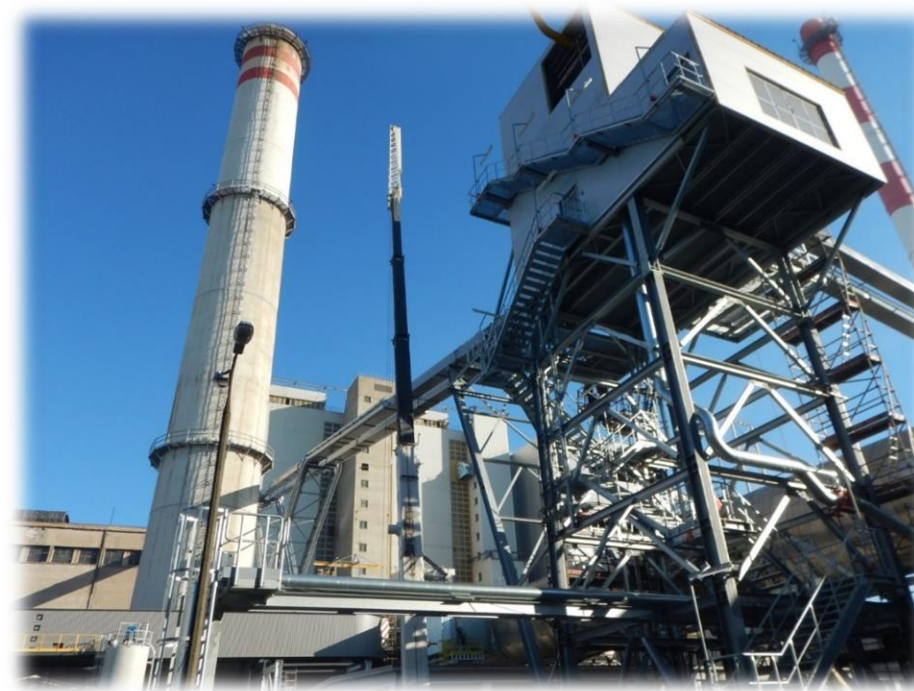
New transfer tower and biomass feeding pipeline
