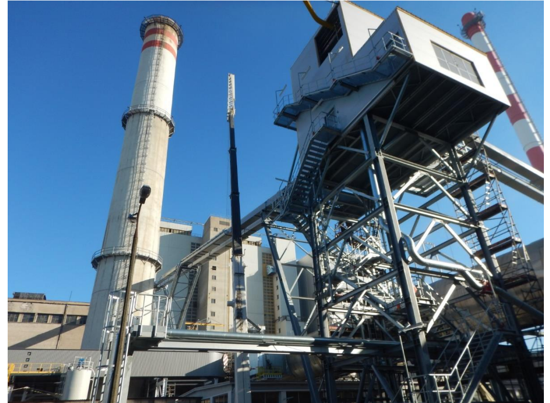
New transfer tower and biomass feeding pipeline
