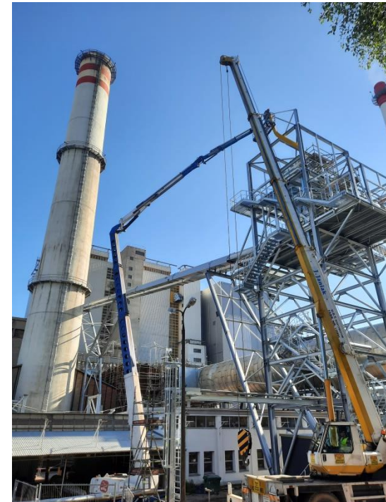
New facilities for the biomass feeding system to K7 boiler - transfer tower and biomass feeding pipeline to the boiler.
